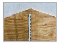
2) Install the nail flange with the factory cut side lined up to the left side of the line you made on your gable.
